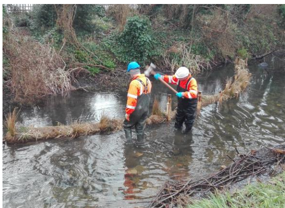
Installing new deflectors in the Lower Duke's River at Riverside Walk
