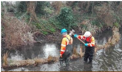
In-stream improvements at Riverside Walk.
