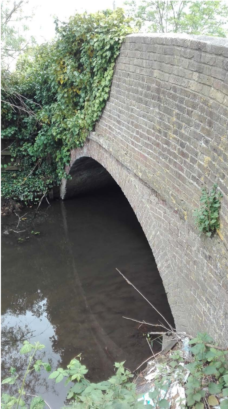
Figure 2: bridge over the Upper Duke's River in Harmondsworth
