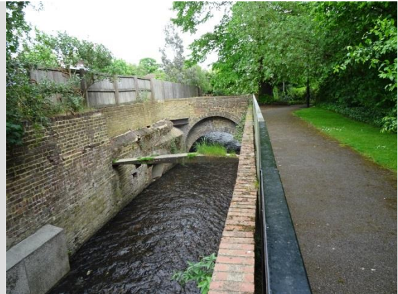
Photograph 4 Brickwork at Watney's bridge
