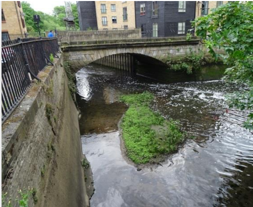
Photograph 3. Mill Platt: possible Daubenton's roost on the Thames- side of the bridge
