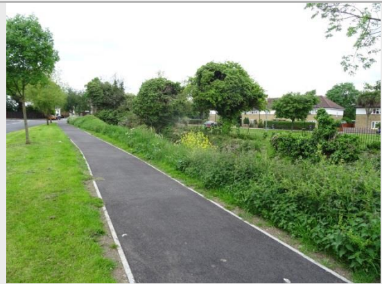
Photograph 2. Removal of trees and new tilted LED lights urbanising the Riverside Walk
